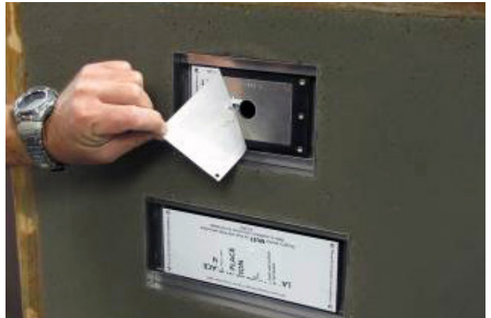
STEP 4 Remove temporary cover plate label.
