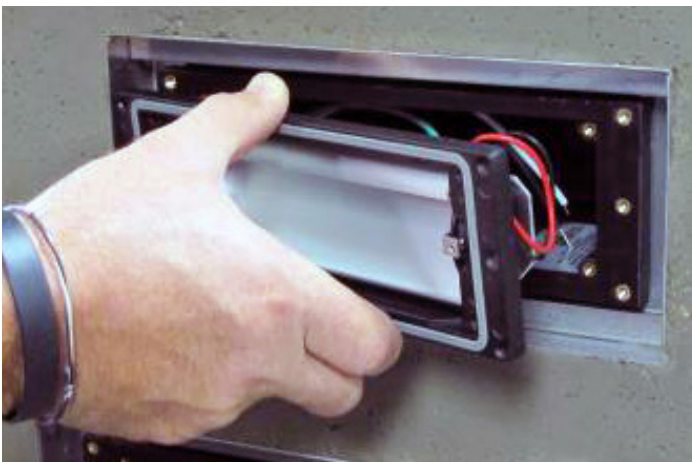
STEP 8 Install Performance Optic Package (PoP).
