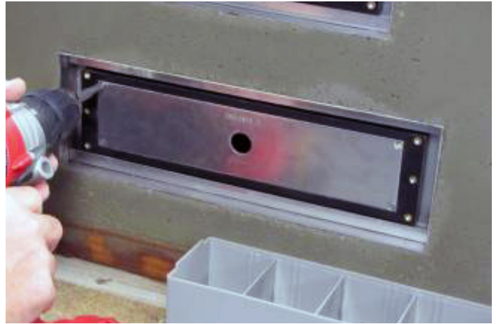
STEP 5 Remove internal support plate.
